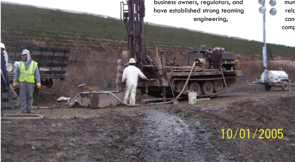
Drilling adjacent to landfill MSE wall
